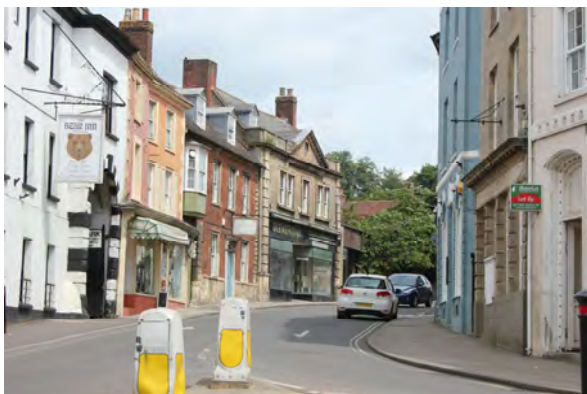
The pedestrian environment is frequently compromised by the highway layout
